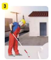
Dilute MONOSTOP PU HYBRID with clean water at a ration up to 10% and apply the first layer with brush or roller. Then let to dry well.
