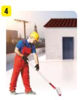
Apply the second layer (without dilution) crosswise after 12-24 hours depending of the weather conditions
