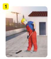
To ensure proper adhesion of the paint, surfaces should be smooth, clean and dry, free from grease, dust, loose or flaking material.
