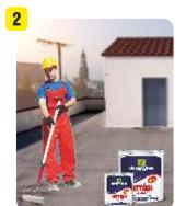
For the stabilization of the substrate and for better adhesion of that, surfaces should be primed with LIFE DUR diluted with White Spirit at a ratio 50%.
